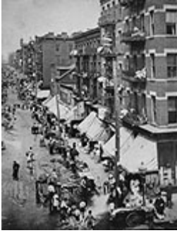
Fig. 1 Orchard Street, View looking south from Hester Street, New York City, 1898
